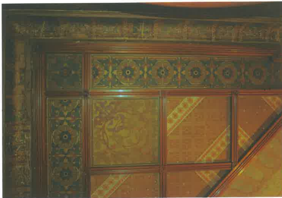
Fig. 12. Company Room D, detail of ceiling following completion of the project, 2012.
