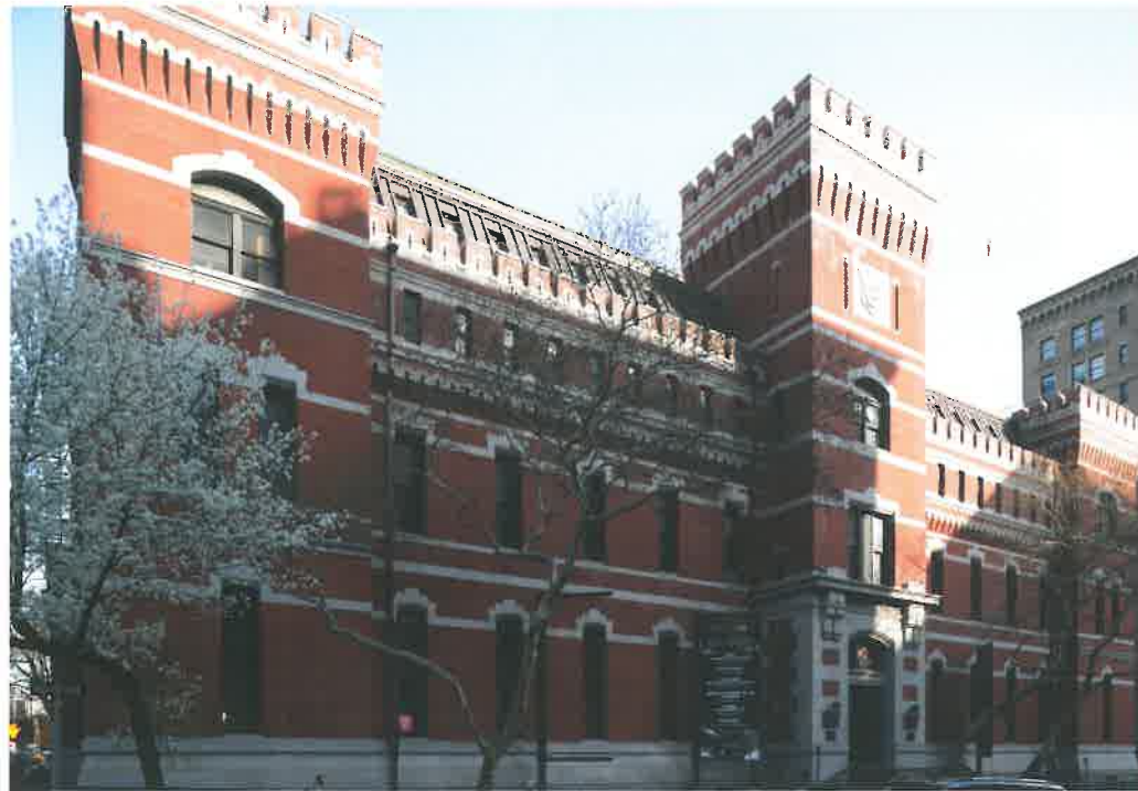
Fig. 2. Seventh Regiment Armory, looking southeast, 2015. All images by Building Conservation Associates unless otherwise noted.
